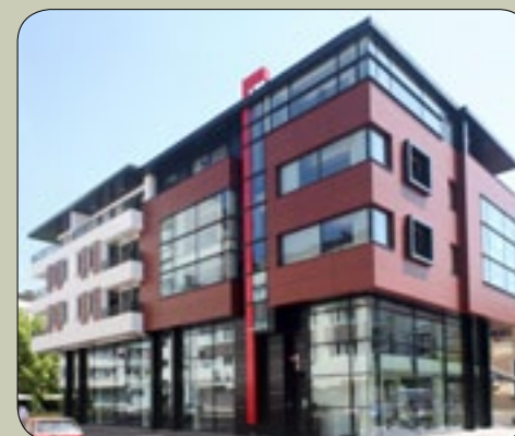
New offices of the Central Registry
